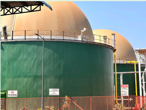
Integrated SWM Facility, Saligao, Goa
