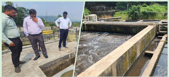
Used Water Management Plant, Lonavala
