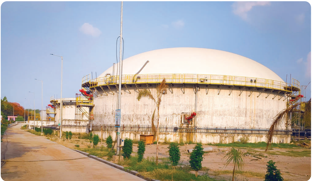
Picture –Typical Digester Design for Anaerobic Process at Prayagraj
