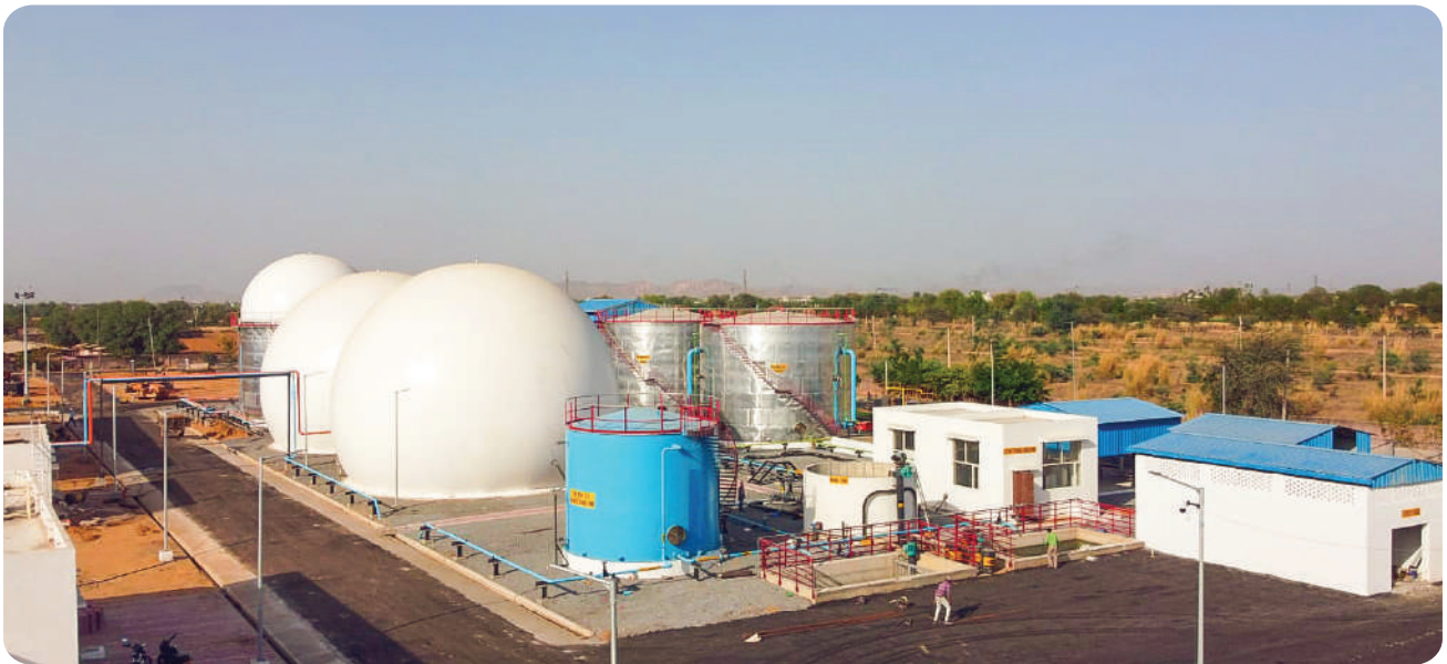
Picture-CBG plant at Hingonia, Jaipur
