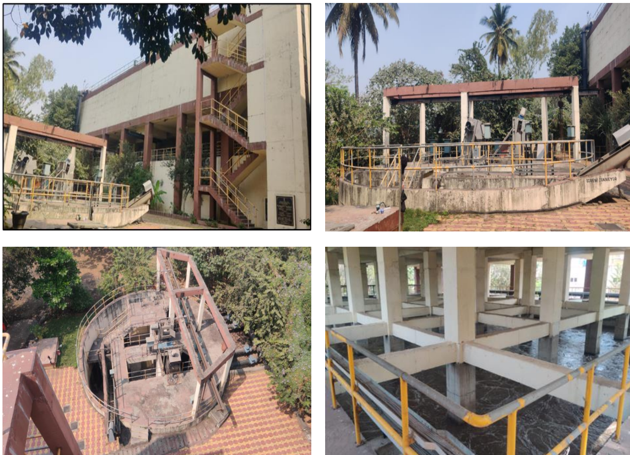
Fig. 3.10: Multi-storey STP in Pune Cantonment, Maharashtra, India
