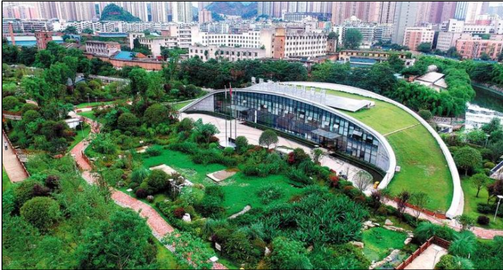
Fig. 4.1: An aerial view of the Qingshan plant, the first underground multi-storey STP in Guiyang, Guizhou Province, China ( https://www.chinadailyhk.com/article/242387 )
