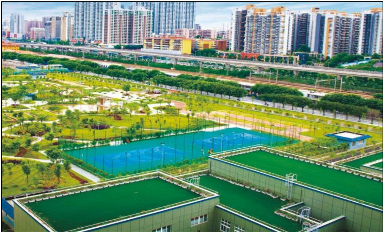
Fig.3.1: Multi-storey STP in Shenzhen Buji, China with a leisure park on the ground ( https://en.ccccltd.cn/yw/dcs/Ecology_and_Environment_Protection/202109/t20210901_142175.html )
