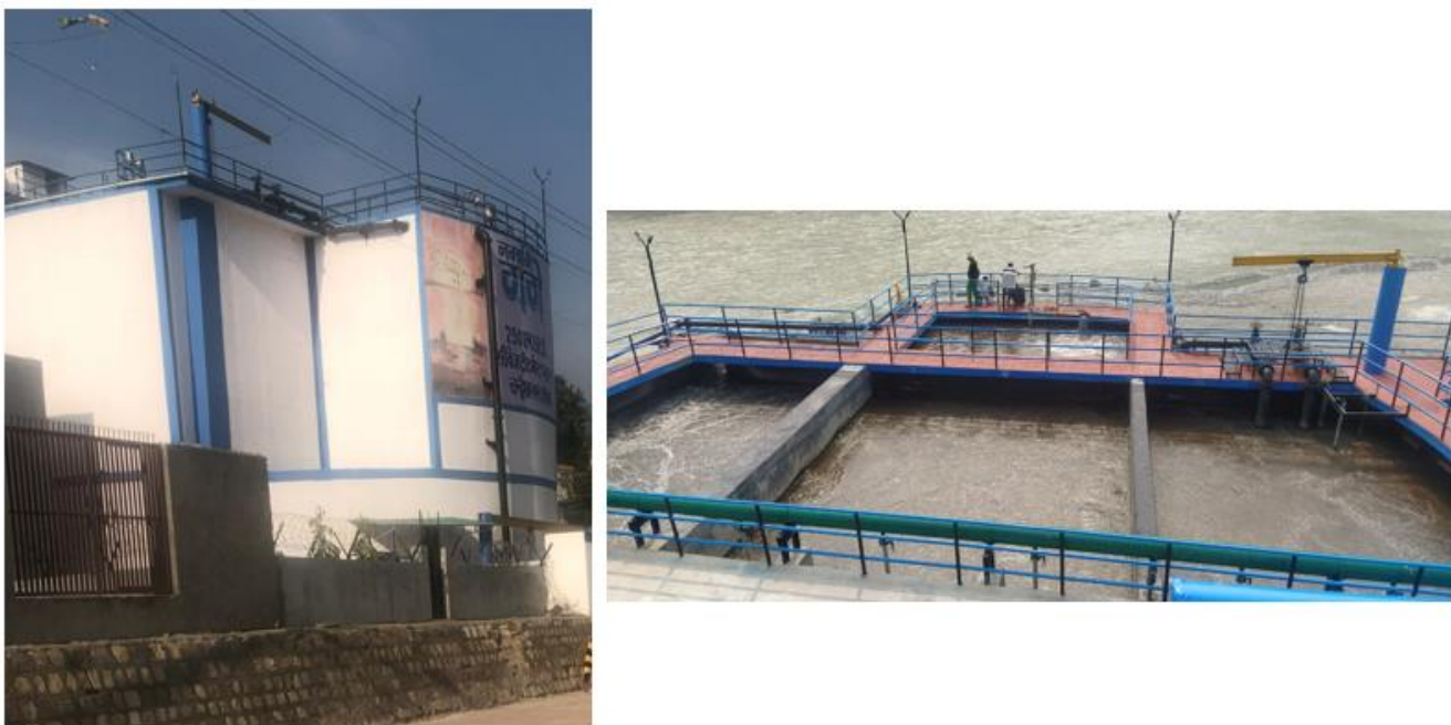
Fig. 3.9: Multi-storey STP in Rishikesh, Uttarakhand, India
