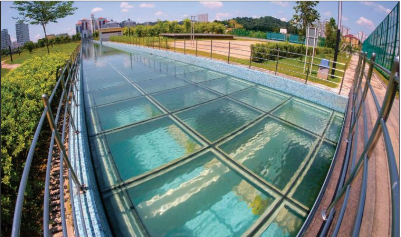
Bio effluent pool provides natural light to the plant below ( https://www.constructionplusasia.com/my/pantai-2-sewage-treatment-plant/ )
