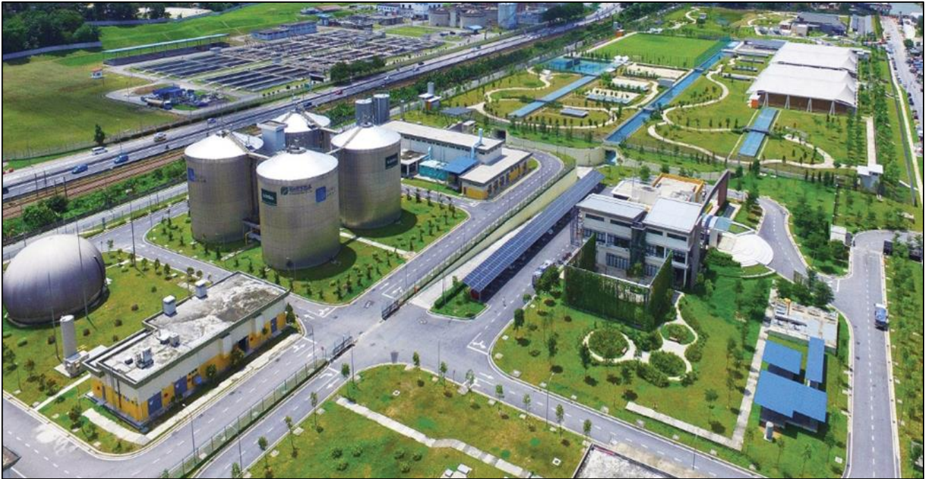
Aerial view of Pantai 2 multi-storey underground STP
