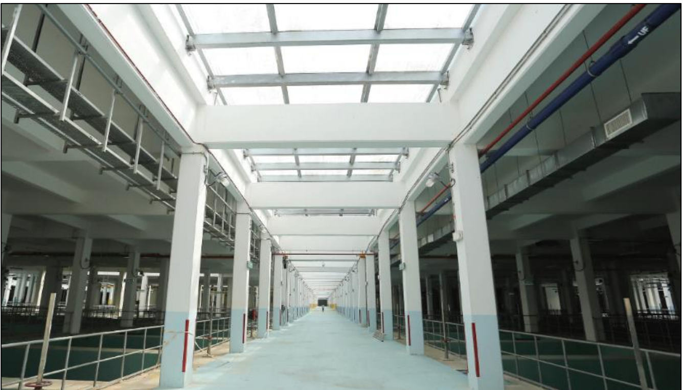
The skylight naturally brightens up the underground plant ( https://www.constructionplusasia.com/my/pantai-2-sewage-treatment-plant/ )
