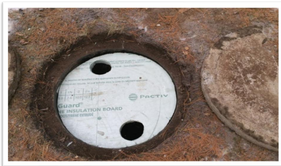
Fig. 4.4: Rigid foam cut to shape concrete Septic Tank cover
