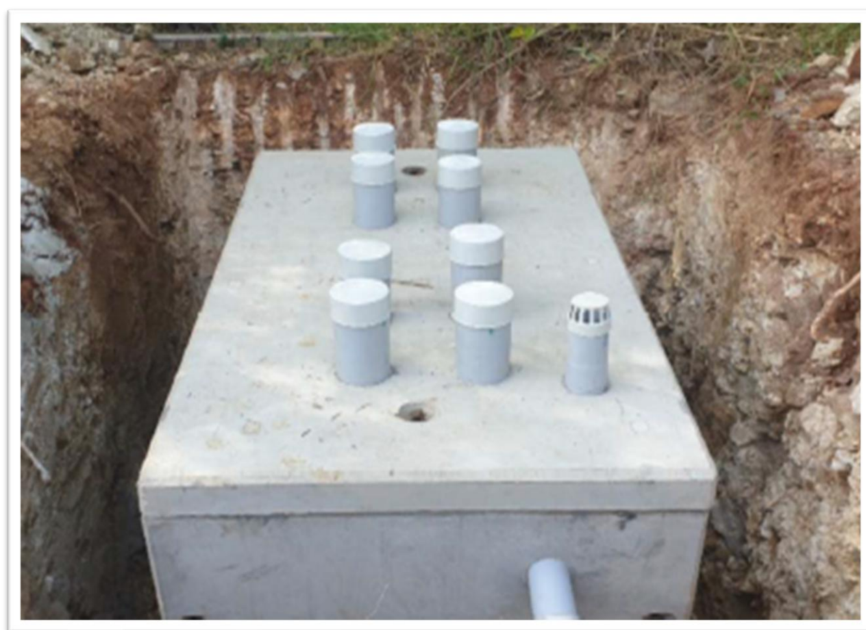
Fig. 3.7: Anaerobic Packaged System with Floating Media
