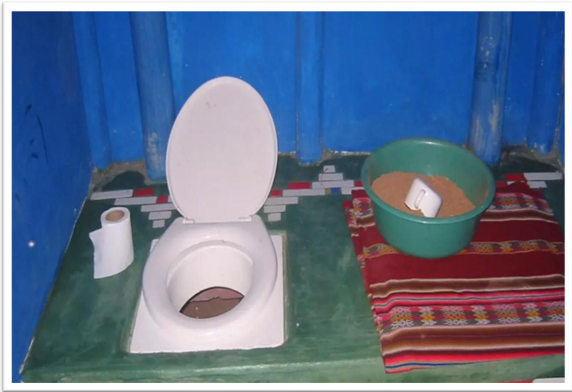
Fig. 3.17: Double Pit Dry Toilet used in Ladakh
