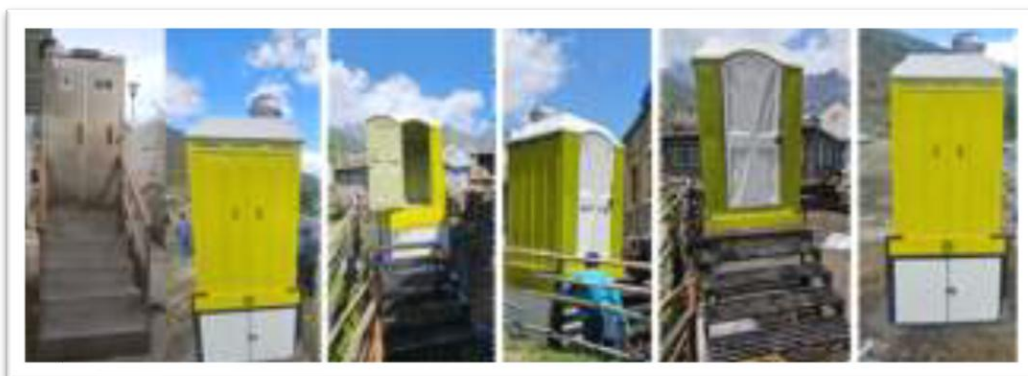
Fig. 1.3: Dry toilet System with Faeces-Urine Separation and Treatment (DToi-FUrST) at CeHAB, CSIR-IHBT, Lahaul
