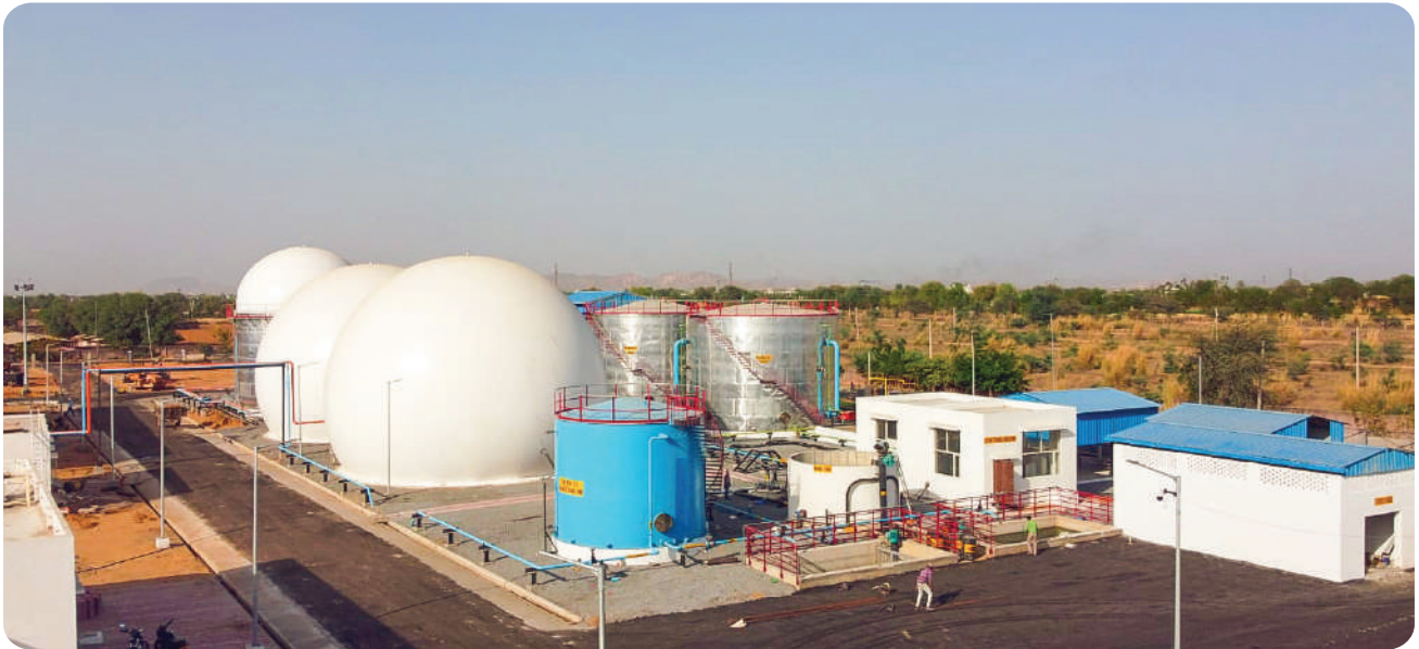
Picture-CBG plant at Hingonia, Jaipur
