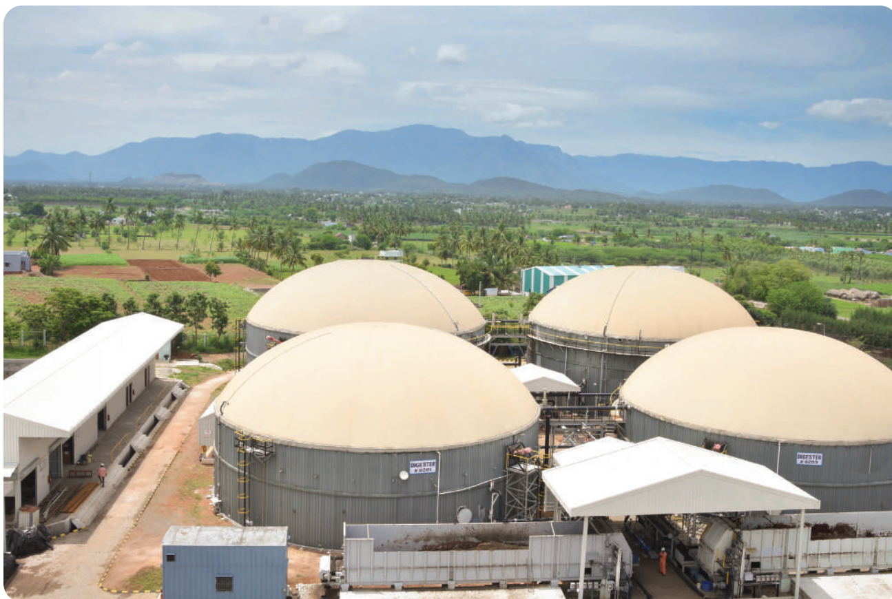
Picture—Fixed-dome Gas Holder at Namakkal CBG plant
