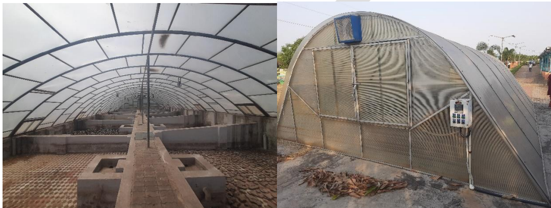
Figure 5.2 SGHD Covered SDBs and On Concrete Platform
