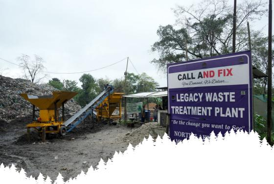
To strengthen ongoing solid waste management, the city generates 36–42 TPD of municipal waste, which is now processed through modern systems. At Japisajia, an integrated Material Recovery Facility (MRF) and Waste-to-Compost (WTC) Plant has been established—Assam's first centre offering recycling, scientific
