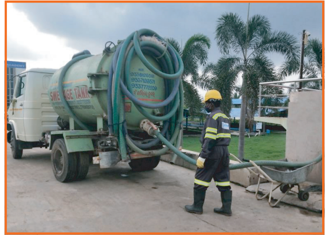
Figure 2 - Mechanical septic tank cleaning
