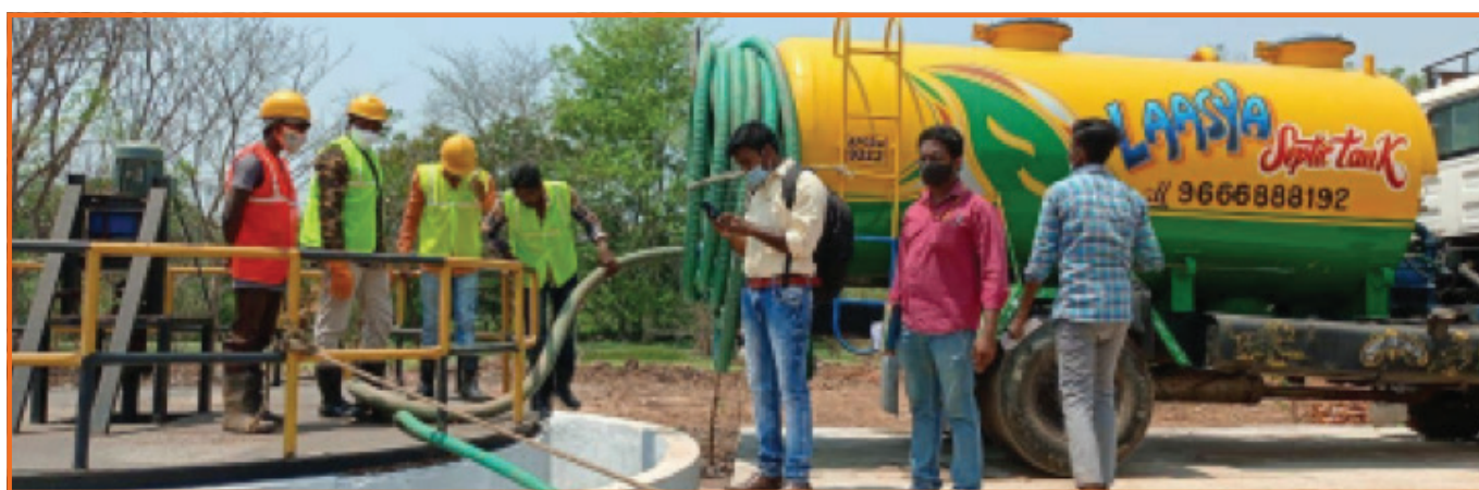
Figure 2 - Periodic desludging
