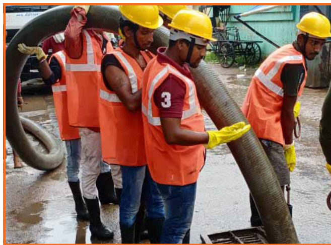
Figure 1.2 - SafaiMitras engaged in mechanised cleaning of sewer lines
