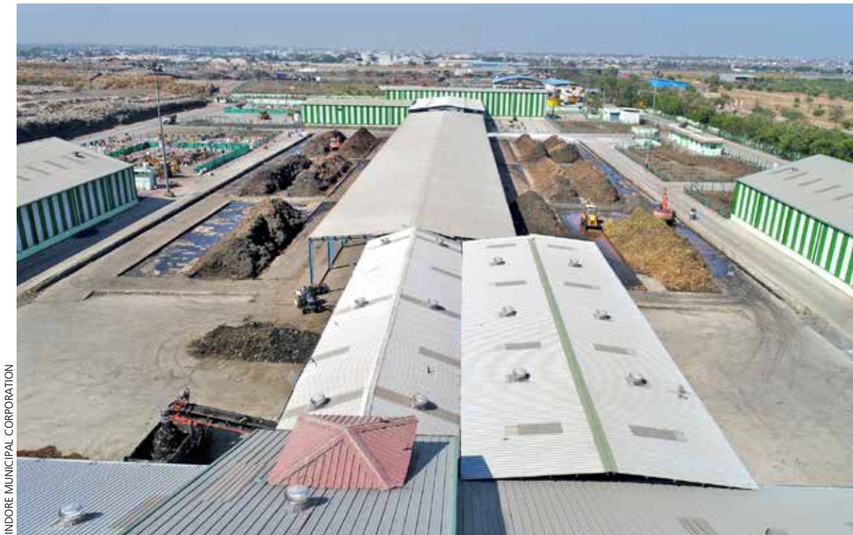
Aerial view of windrow composting in Devguradia
