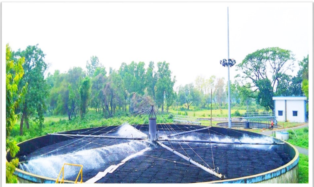
Figure 29: 10 MLD STP with trickling filter at Kalyani West Bengal
