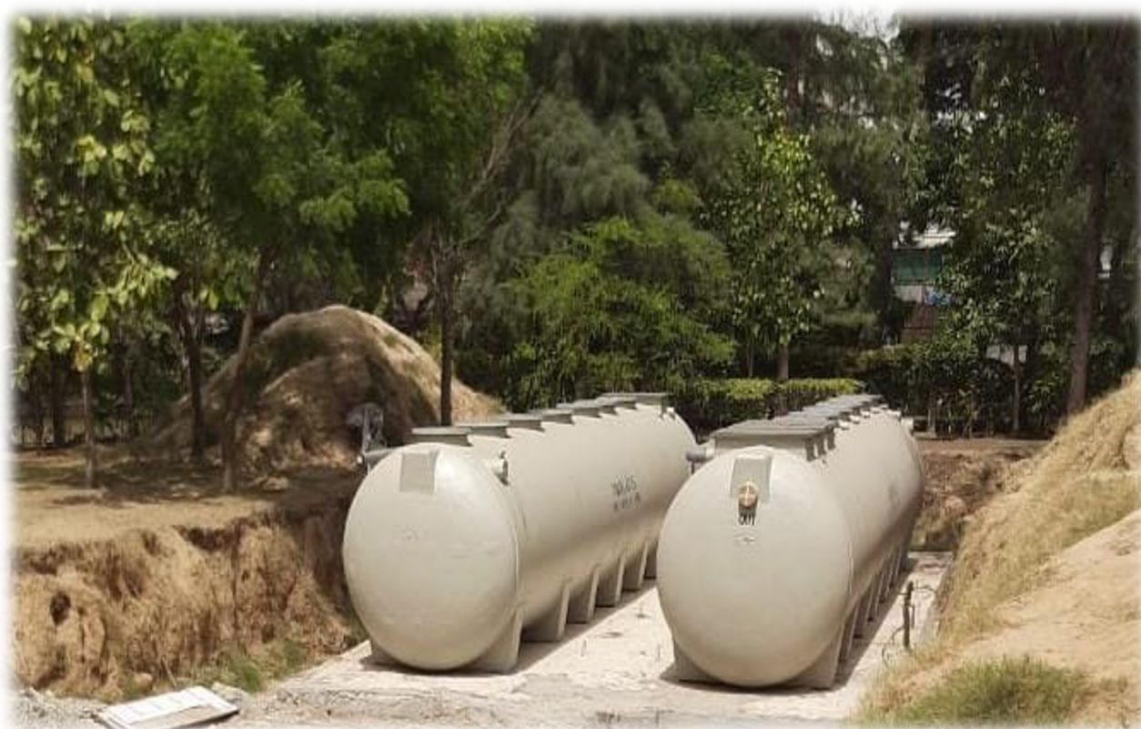
Figure 73 Pre-fabricated Johkasou treatment unit installed in New Delhi
