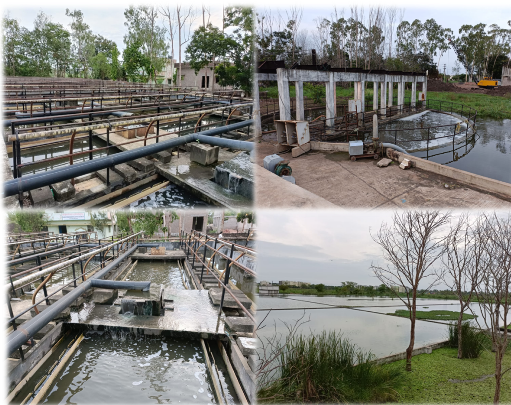
Figure 69 UASB technology based STP installed in Rajamundry, Andhra Pradesh
