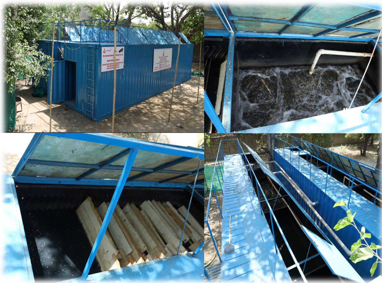
Figure 74 Package sewage treatment plant installed in a residential complex in New Delhi
