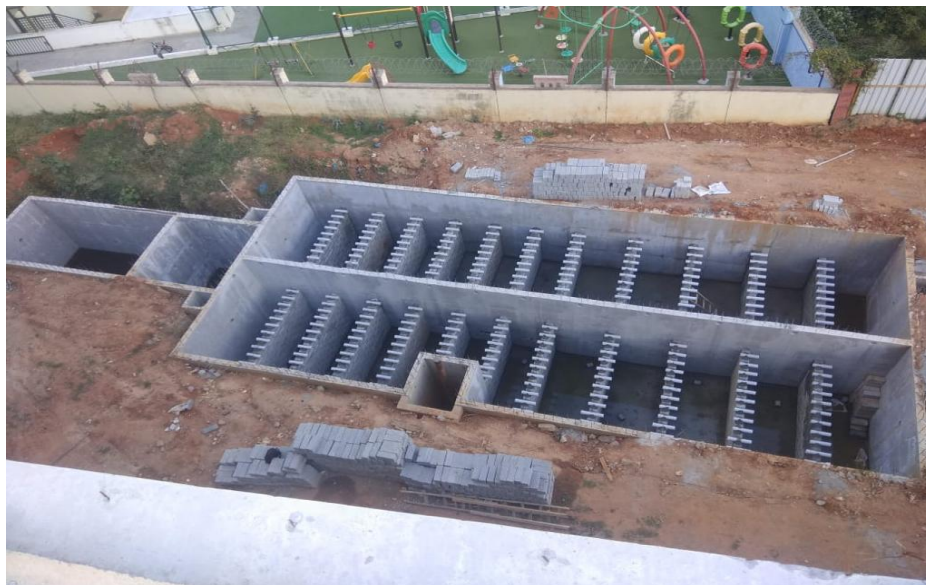
Figure 45 Construction of DTS
