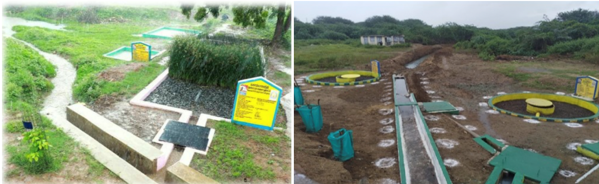
Figure 56: Photograph of Community Soak pit Horizontal & Vertical Filter Type at Tamil Nadu
