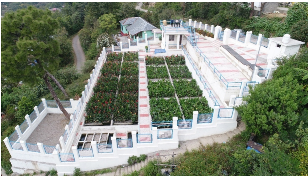
Figure 13: Photo of Root Zone technology based STP (180 KLD STP at Dharamshala, H.P.)
