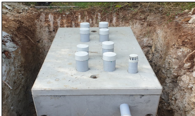
Figure 49: Photograph of Modular DTS being installed in Discovery village Bangalore
