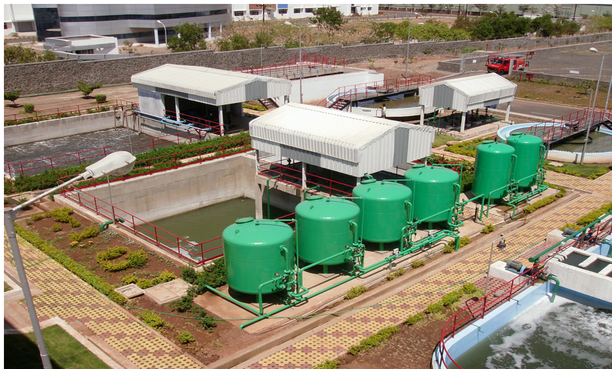
Figure 20: Photographs of Extended Aeration based STP
