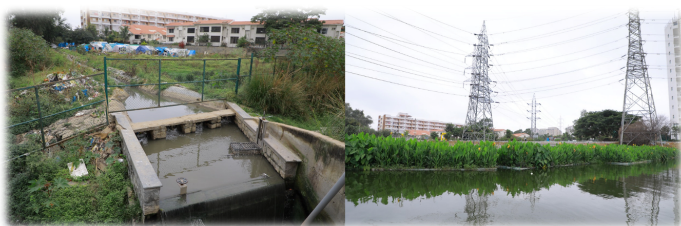
Figure 65 Screen with grit collection structure (left) floating wetlands (right)
