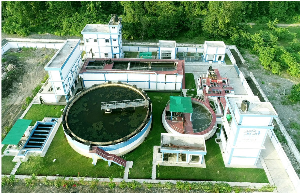
Figure 30 MBBR technology based 5 MLD STP at Uttarakhand
