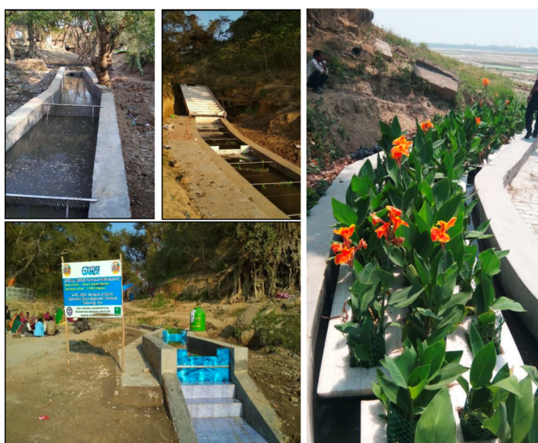
Figure 52: Photographs of the nature-based treatment 12 MLD at drains in Prayagraj
