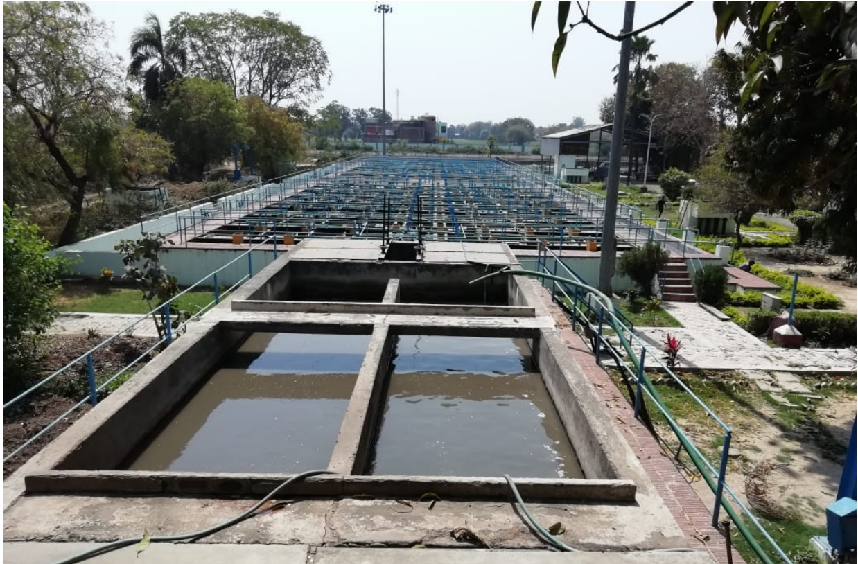
Figure 33: Photograph of 14 MLD UASB technology based STP at Mirzapur, Uttar Pradesh
