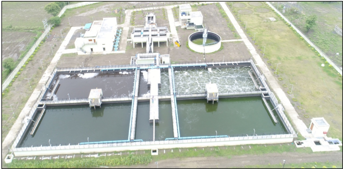
Figure 23: SBR based STP
