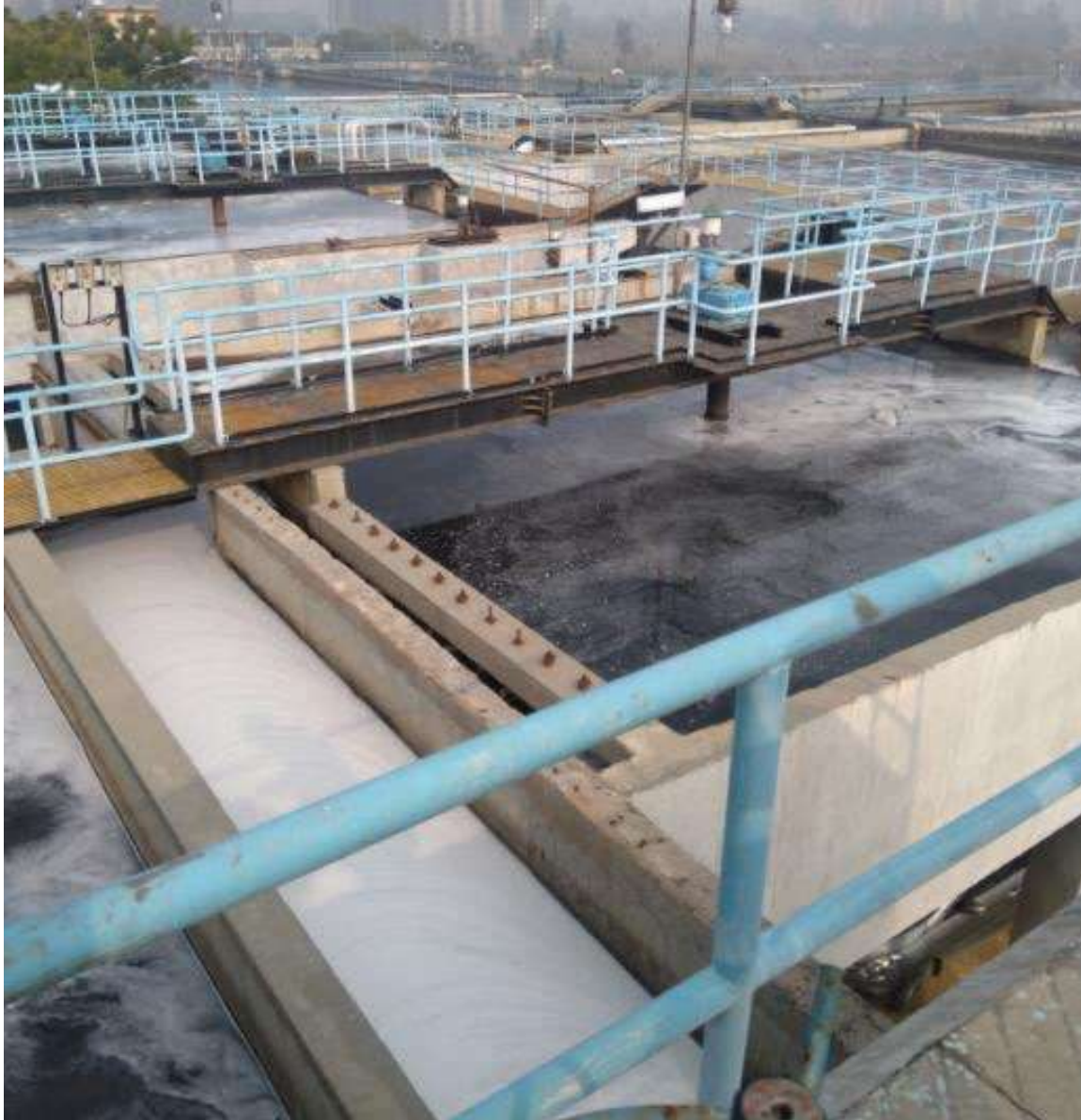
Photograph of STP plant
